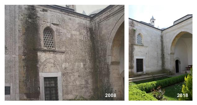
Figure 6 - Before (2008) and after (2018) facade cleaning.
