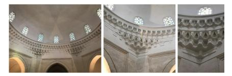
Figure 18 - Muqarnas used in spaces with their acoustic properties.
